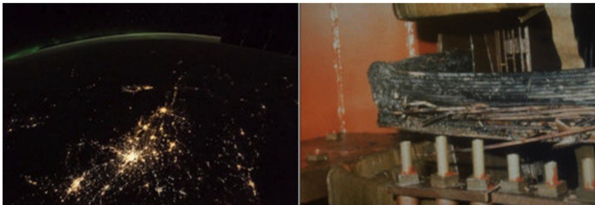
A power blackout (left) and transformer damage (right) during the March 1989 storm.
