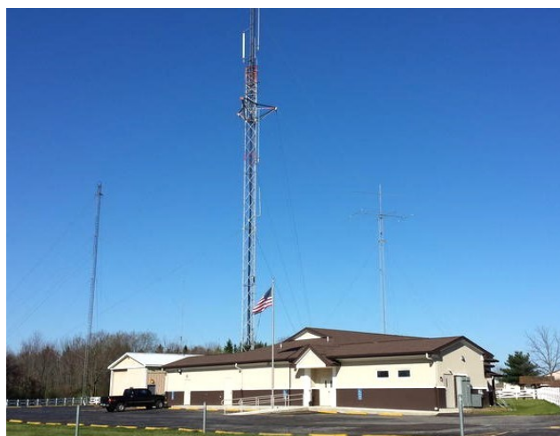
DARA Clubhouse & Antennas
